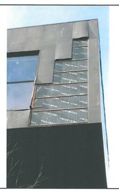
Photo of copper paneling that is damaged and coming loose from the building
