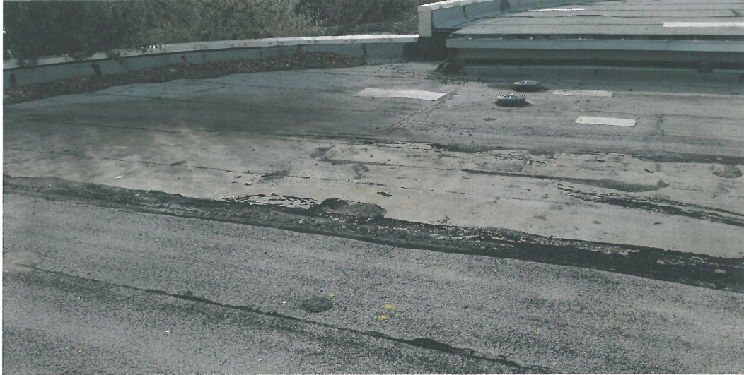
View of Lamb roof condition: Shows patches, cracks, and alligator marks on the roof.
