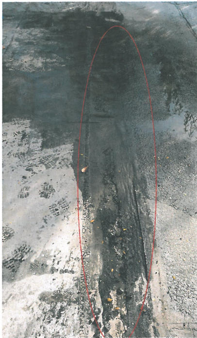
Major leak on roof Shows where the roof has completely cracked and exposed the under coating. Results are major leak in the middle of the library.
