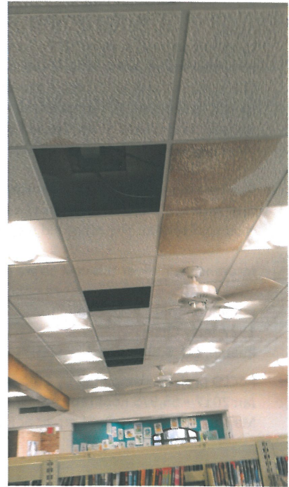
Major leak on roof Shows where the roof has completely cracked and exposed the under coating. Results are major leak in the middle of the library.
