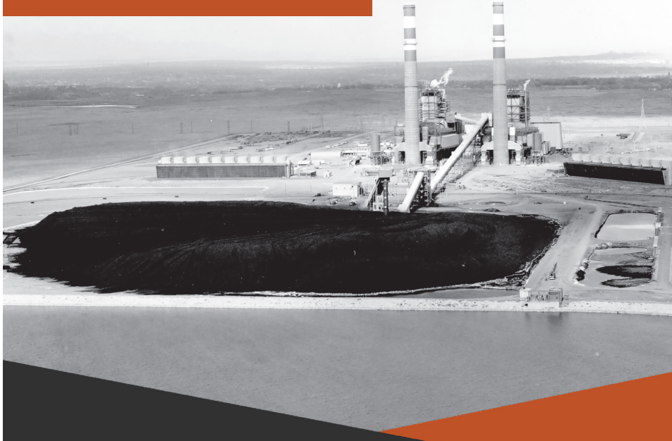
Comanche coal-fired electrical generating facility
