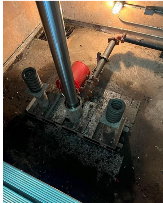
30. View of pit with cylinder, piping, and spring buffers.
