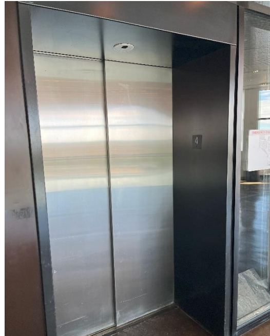
18. Typical elevator entrance with Braille in jamb.
