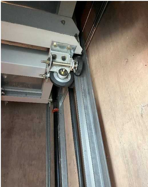
31. Bottom of car roller guides.
