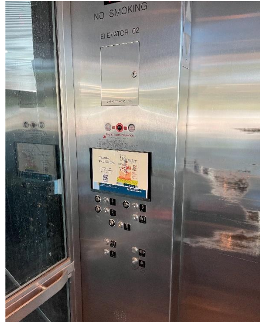
2. Elevator 2 car operating panel with locked service cabinet and hands-free communication device.
