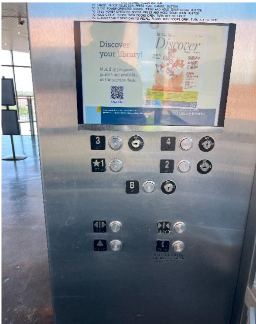
15. Car operating panel with keyed access switches and hands-free communication device.
