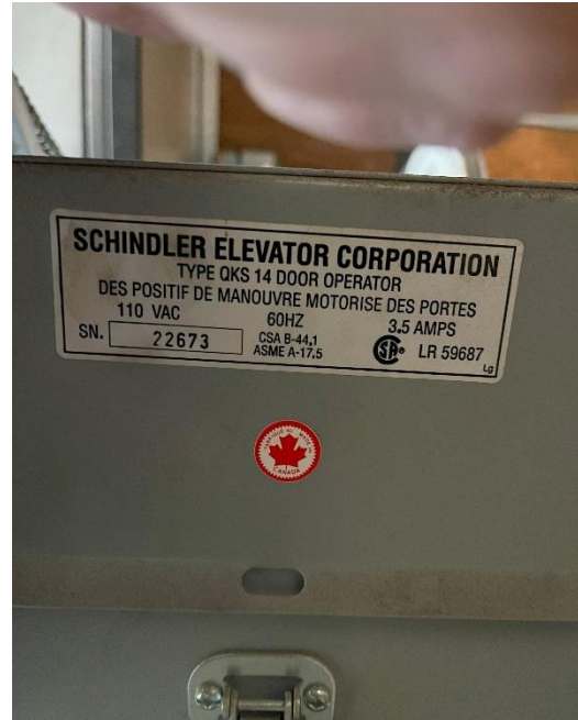
42. Data tag for Schindler door operator.
