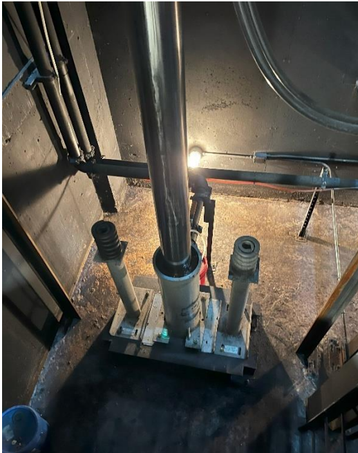
9. View of pit with hydraulic cylinder, piping, and spring buffers.
