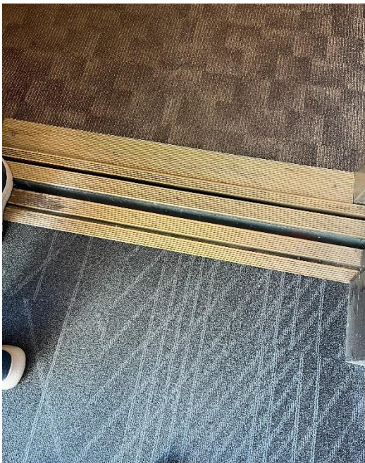
23. View of car and hoistway sills.
