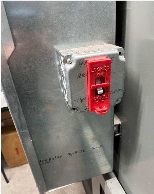
5. Power switch for car top workstation.
