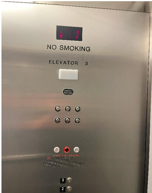
25. Car position indicator with keyed access switches in elevator 3.
