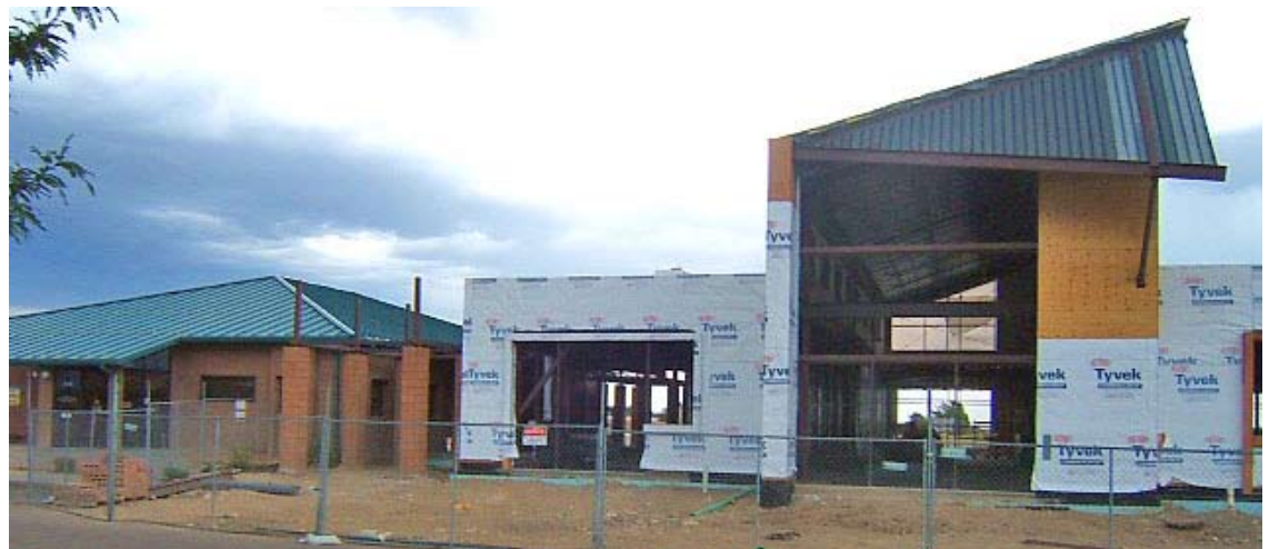
Library patrons are excited about the nearly 25,000 square foot addition to the Pueblo West Library.
