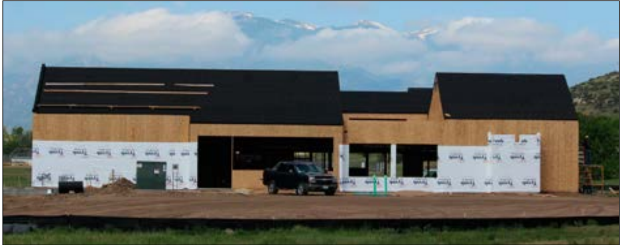
Construction progress on the new Greenhorn Valley Library.
