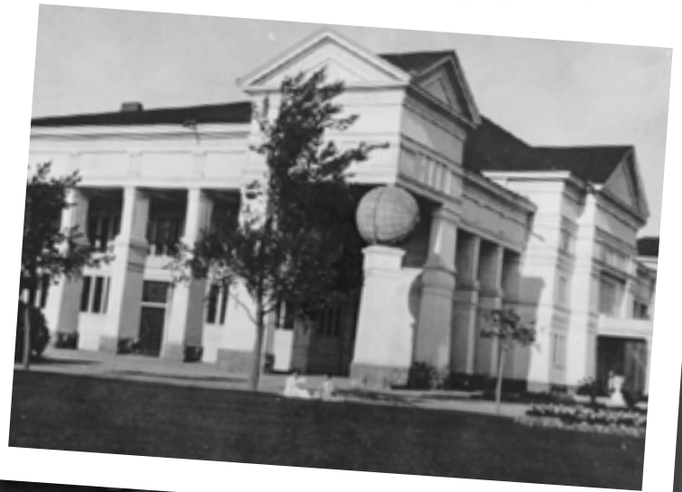
Mineral Palace exterior.
