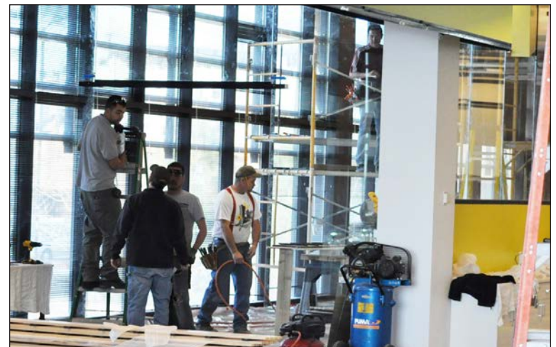
Construction workers install glass in the Idea Factory, a space to explore and create.
